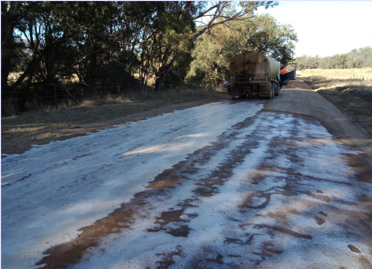
Surface application of Polychlor Omega for dust suppression. After 10 minutes, the road can be reopened to traffic.
